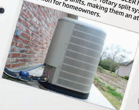
Long found in mini-split systems and window units, inverter-driven rotary technology is now finding a home in traditional duct systems too.
